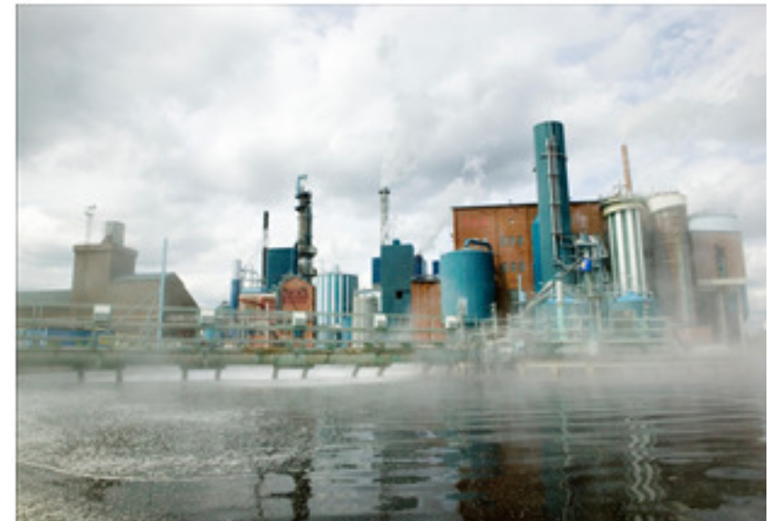
Location of one of the Swedish projects: Rottneros Vallvik pulp mill
