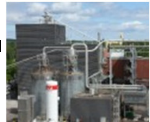
StoraEnso Pilot Plant
