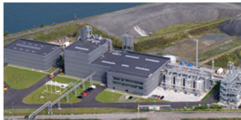
Inbicon Biomass Refinery at Kalundborg
